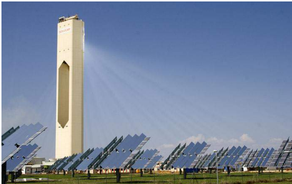
P10 Solar power plant, Andalucia, Spanje
